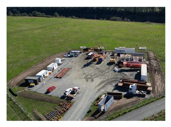
Work is well underway on the new water supply pipeline for Wingham, with crews currently drilling under the Manning River at Bootawa. This replaces the original 1960s trenched pipeline that was damaged in the May flood. Since then, water to Wingham has been supplied through the Taree town network.
